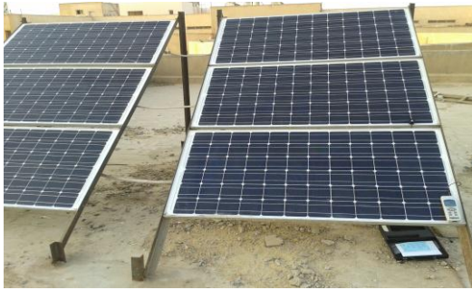
Figure 11: Installation of PV array
