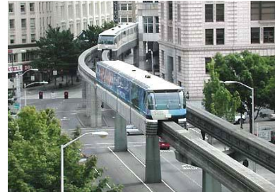
Figure 3.1: Seattle Alweg Monorail, Straddle Monorail (1962). Source: (Kennedy, Considering Monorail Rapid Transit for North American Cities)
