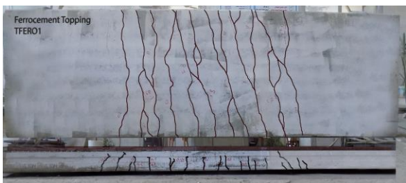
Fig.18: Crack patterns, crack distribution and failure mode for specimen TFERO1
